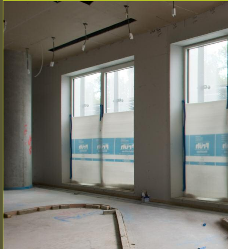
Specifically designed for protection of curtain walling/glazing
